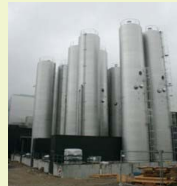
New plant scheduled to be operational in September
