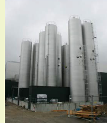
The new Milei GmbH plant under construction
