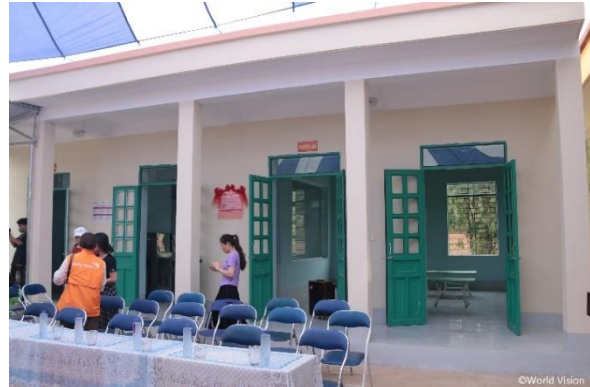
The new kitchen facility in the kindergarten
